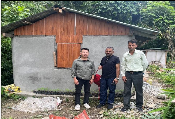
Inspection of PMAY-G house at Taza GP
