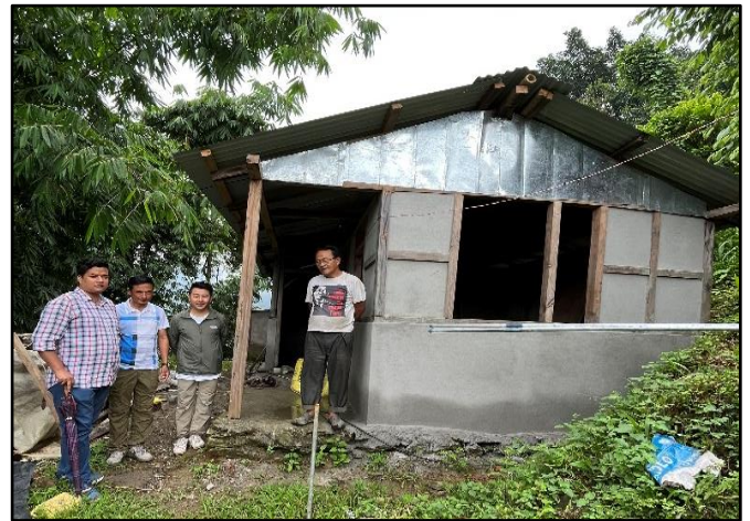
Inspection of PMY-G house at Namcheybong GP
