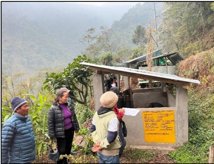
Inspection of Pigshed at Samdong Kambal GPU
