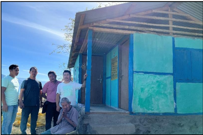
Inspection of PMAY-G house at Rumbuk GP
