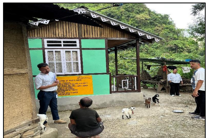
Inspection of PMAY-G House at Sangadorjee GP
